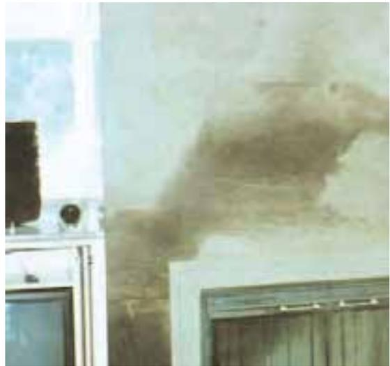
*Wet stone on granite fireplace from a leak in chimney.*
